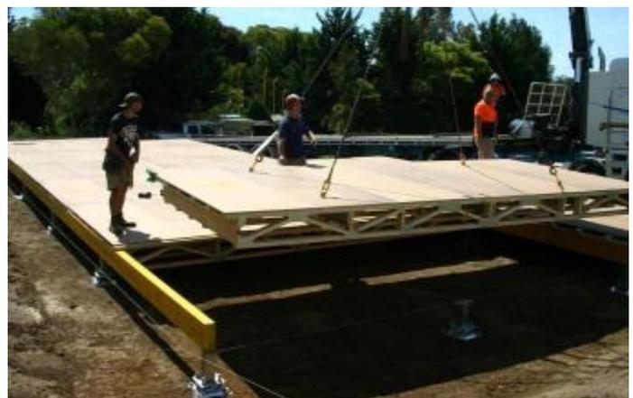
*Drouin West Timber and Truss installed their prefab timber floor on a house site at Corinella in just two days.*
