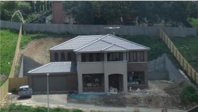
*Concrete slabs aren't always appropriate. Here excavation and retaining wall costs were significant and the functionality and usability of the house block is now clearly questionable.*
