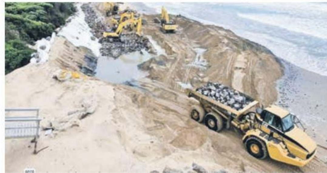
In 2021, the State Government invested $7.6 million to address erosion problems at Apollo Bay, with works including sand-covered rock reinforcement on the foreshore. Why not at Inverloch?
